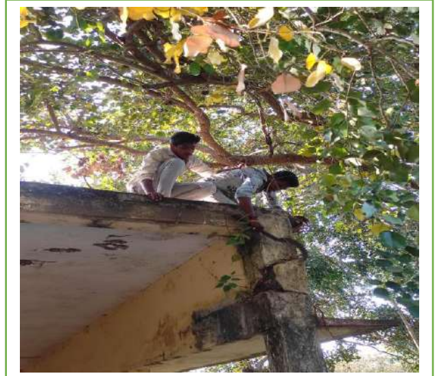
Removing Sacred fig that went deep into the walls
