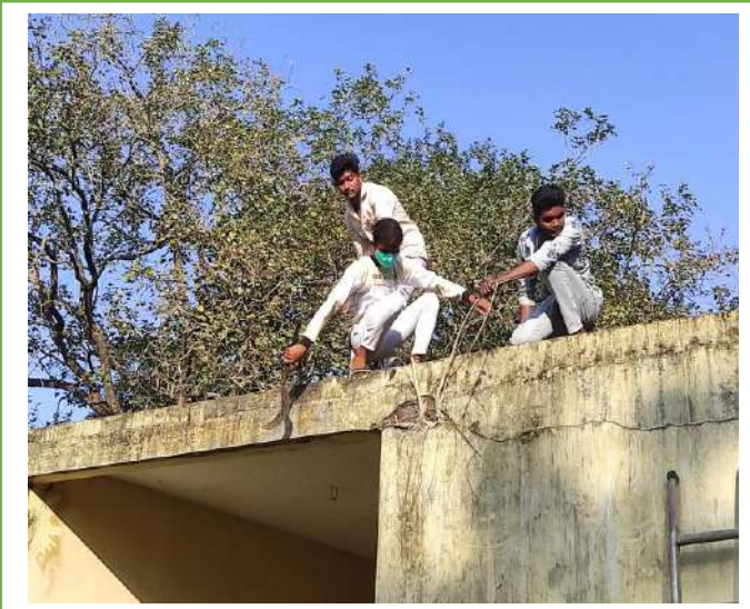
Removing Sacred fig that went deep into the walls
